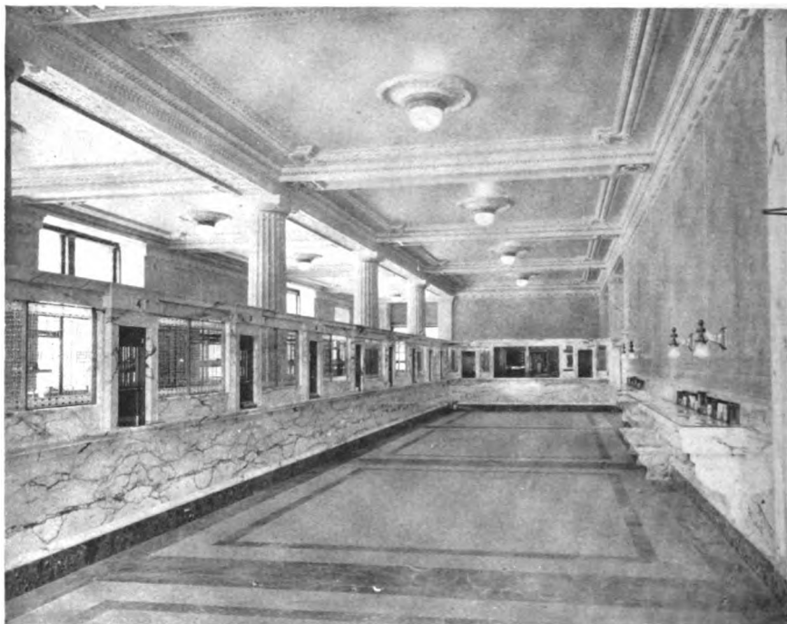
WEST LOBBY AND RECEIVING WINDOWS
